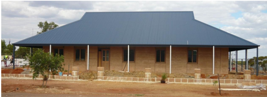
Above – house funded by Shire nearing completion
