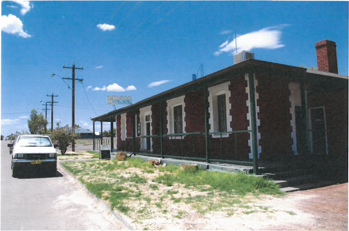
The front of Yalgoo Hotel lacks seating & trees but is also a blind spot for the publican
