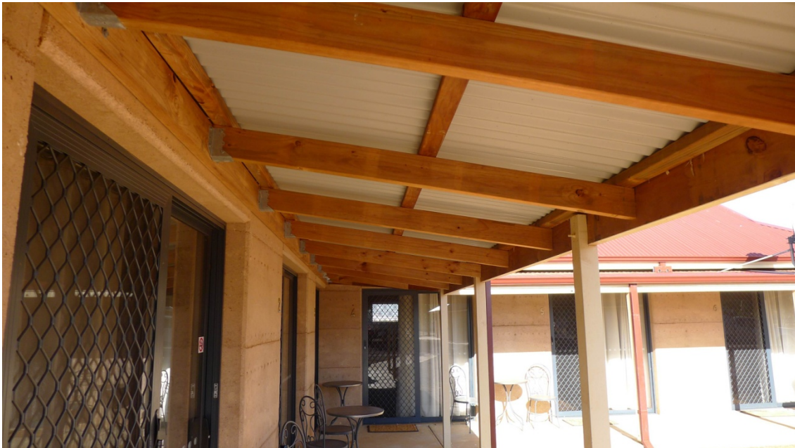
Eaves detail showing lean to verandah, exposed unpainted rafters and bird boards verandah posts, sliding doors.
