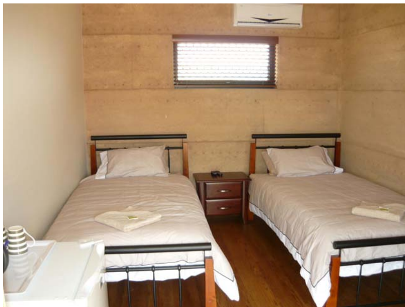
Typical interior (bedroom) showing selected vinyl plank floorcover, off form sealed rammed earth walls, painted plaster lined stud wall.
